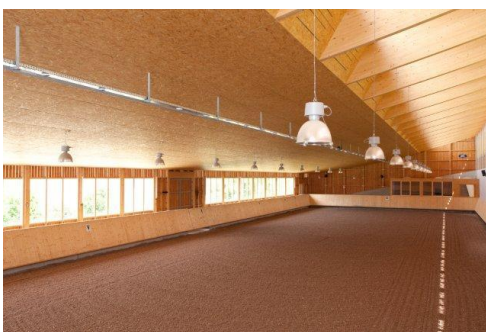
This indoor equestrian arena at the Marbach stud farm was largely built with wood-based materials from KRONOPLY.
