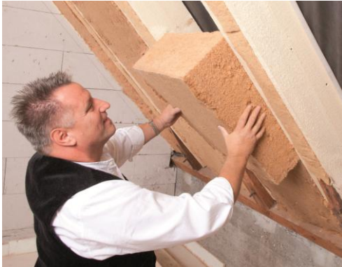
Harald Sauter, a master carpenter and KRONOTHERM application technician, demonstrating the use of KRONOTHERM flex wood-fibre insulation.
